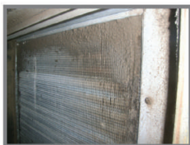
Mold & bacteria on a filter
