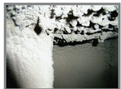
Mold & bacteria in a duct
