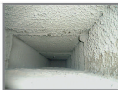
Mold & bacteria in a duct
